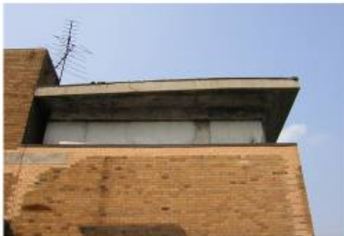
BEFORE: The tower had been boarded up for years
