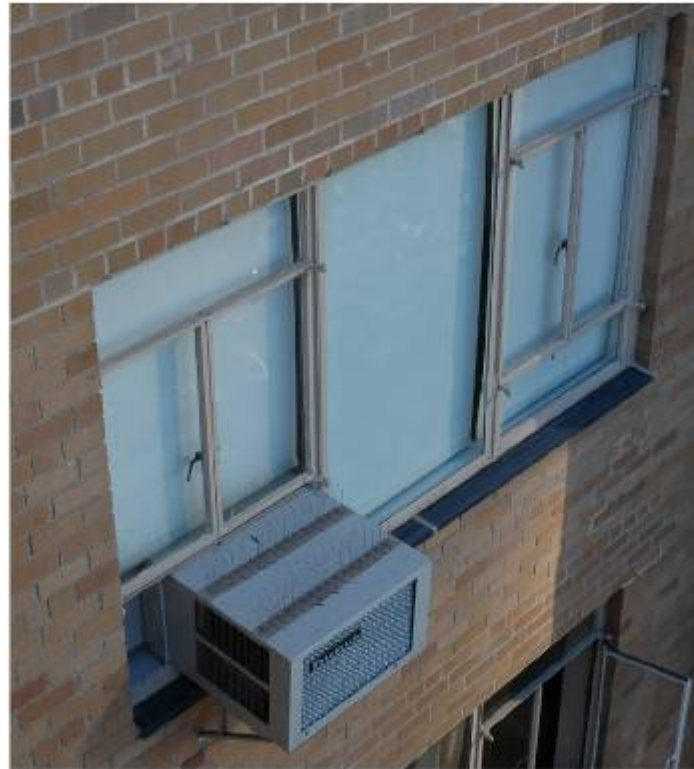
AFTER: All slate sills were replaced, lintels were replaced or repaired, windows were recaulked and painted.
