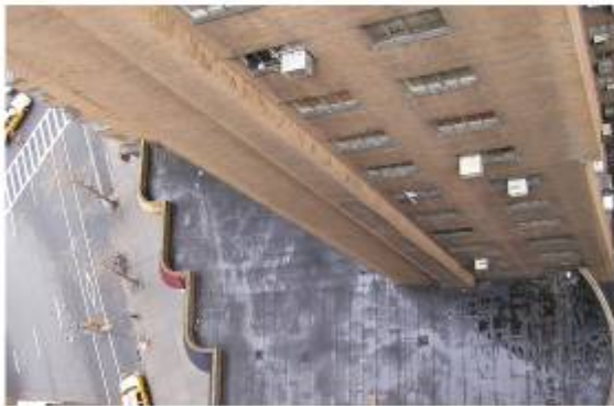
BEFORE: The planters were removed, leaving a blank asphalt roof.
