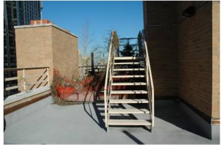
AFTER: Obsolete ductwork and equipment were removed throughout the building.
