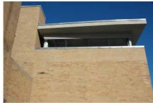
AFTER: Lighting was restored behind a new glass enclosure
