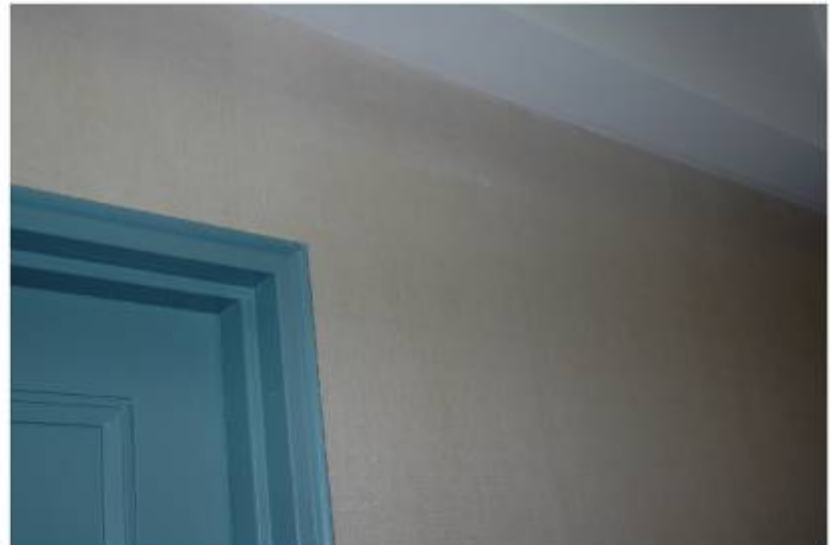
AFTER: New cables, electrical conduits and telephone lines were installed throughout the building and hidden behind newly installed soffits below hallway ceilings.
